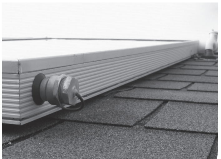
INSTALLING THE ROOF SENSOR
