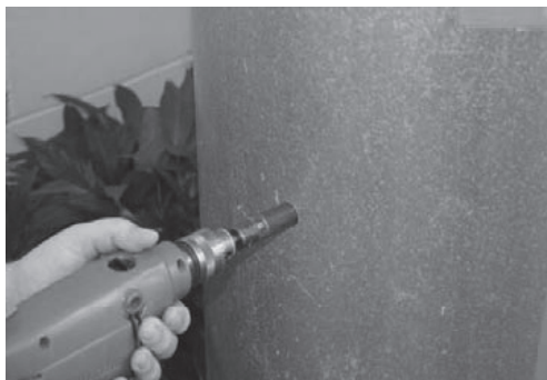
DRILLING 18MM HOLE
